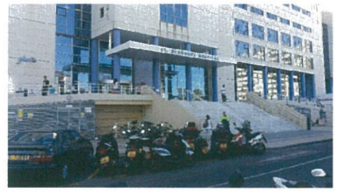
Photo 2: Existing Steps to Main Entrance
